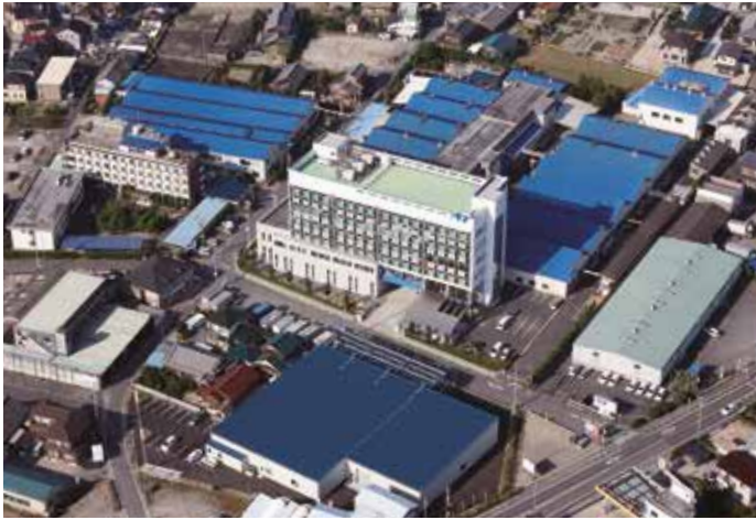
SEDE CENTRAL - HEAD OFFICE
